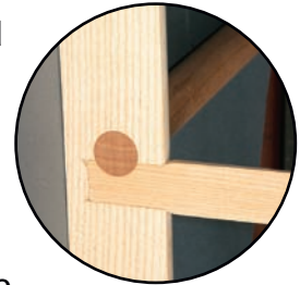
interlocking dowel joints
